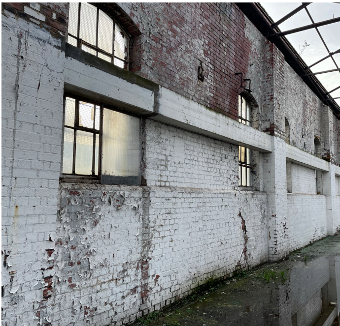
Existing condition of the wall - northern face
